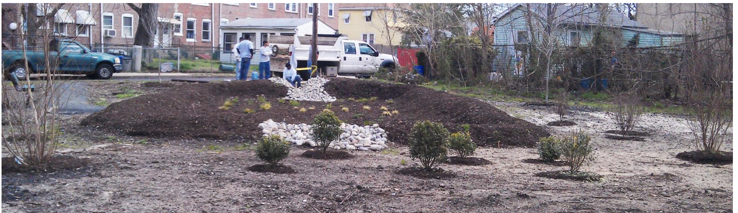
A 900 square foot rain garden in Gloucester City with native trees and shrubs for perimeter landscaping.
